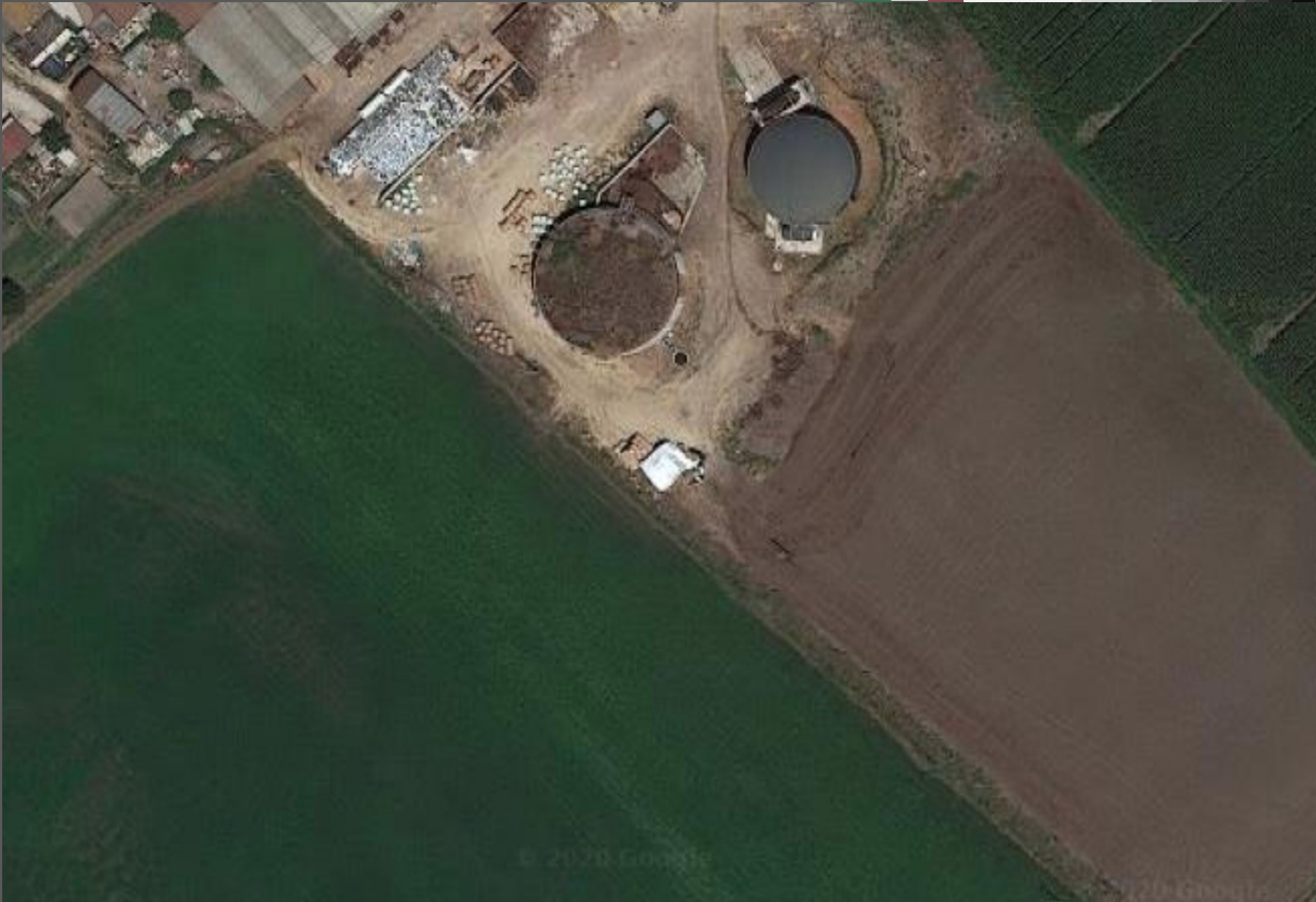
Biogas - Pontinia (LT), Italy - P=250 kW
